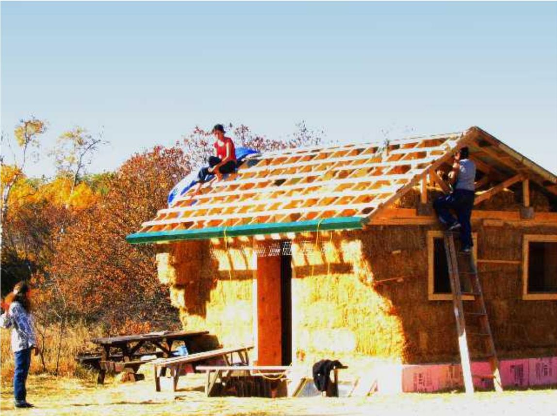
**Figure 2: *The Loo With A View* - Roofing the load-bearing strawbale structure at Brightwater Science and Environment Centre. Pictured from left to right: Carol Vandale, Alison Ledoux, and Stephanie Whitehead.**
